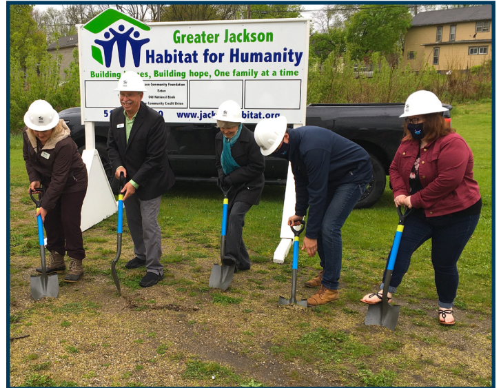
Groundbreaking for the DeLand Pointe housing development.
