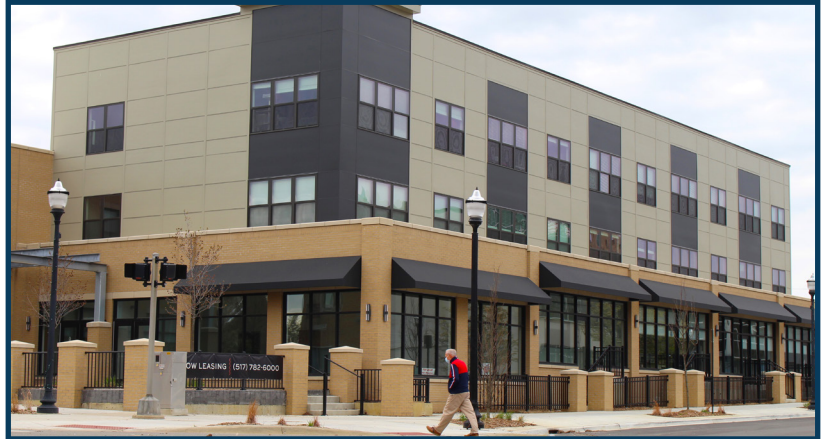
New section of the Albert Kahn Apartments on S. Jackson Street.
