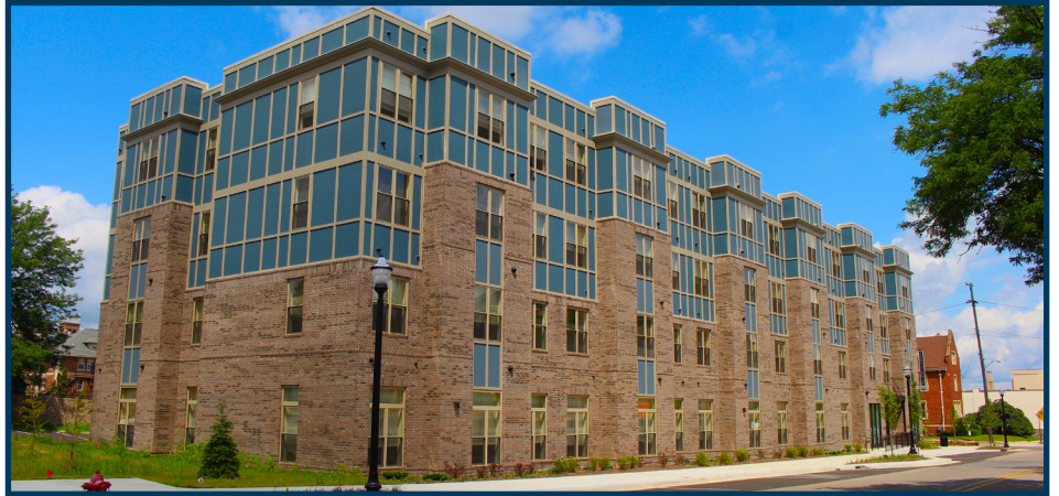
The newly constructed Francis Senior Lofts on S. MLK Drive.
