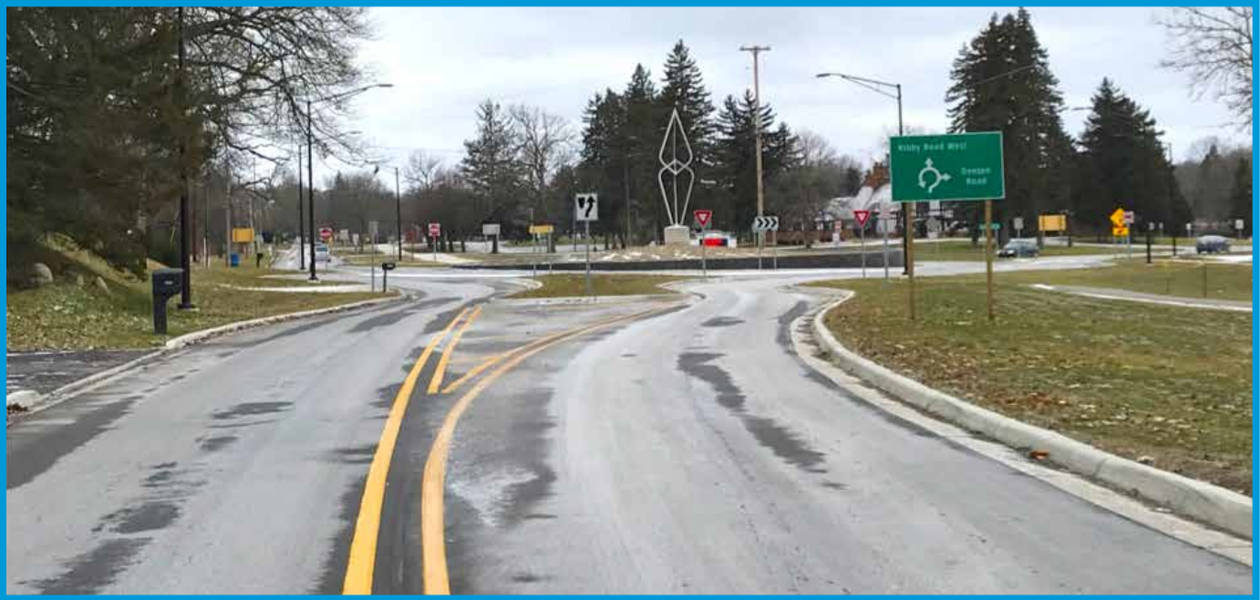
ABOVE: Completed Kibby Road roundabout and street redesign.
