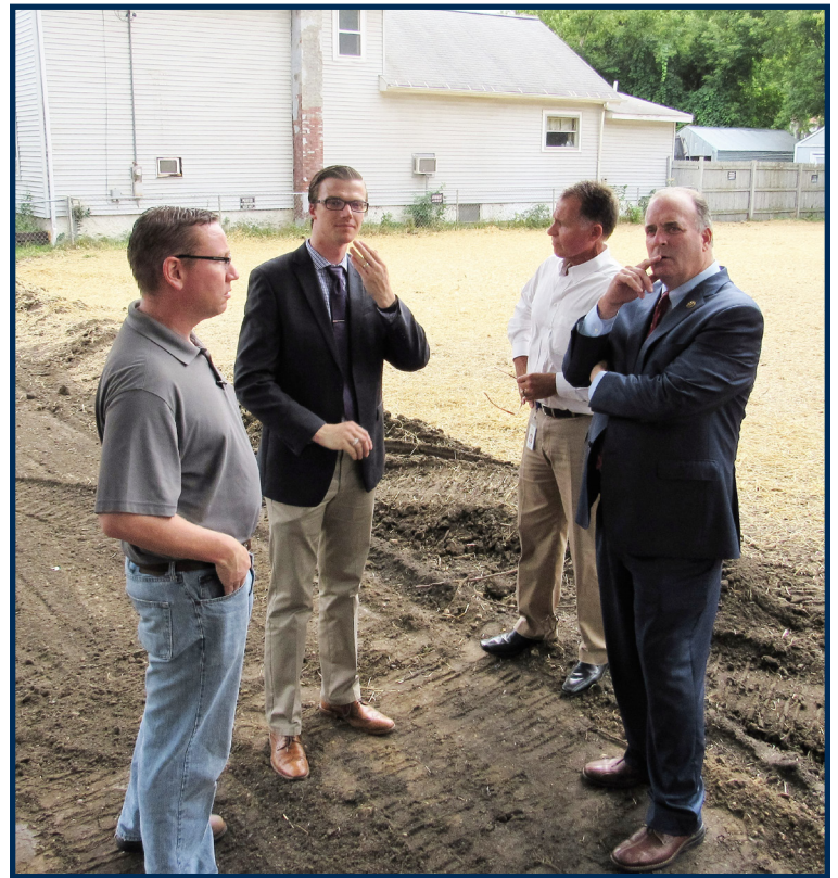
From left to right, Councilman Andrew Frounfelker, Councilman Derek Dobies, City Manager Patrick Burtch and U.S. Representative Dan Kildee tour a City demolition site.
