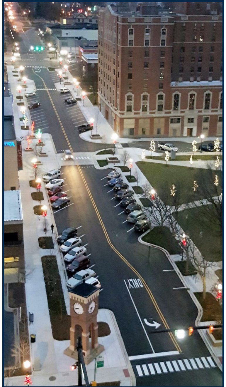
Cars and Christmas lights line the newly constructed Michigan Avenue in downtown Jackson.
