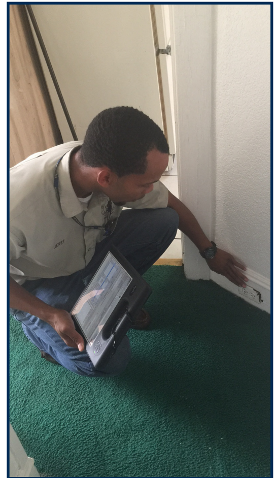
Code enforcement officer Jerry Stackhouse oversees construction work on a Jackson apartment. deadline accordingly."
