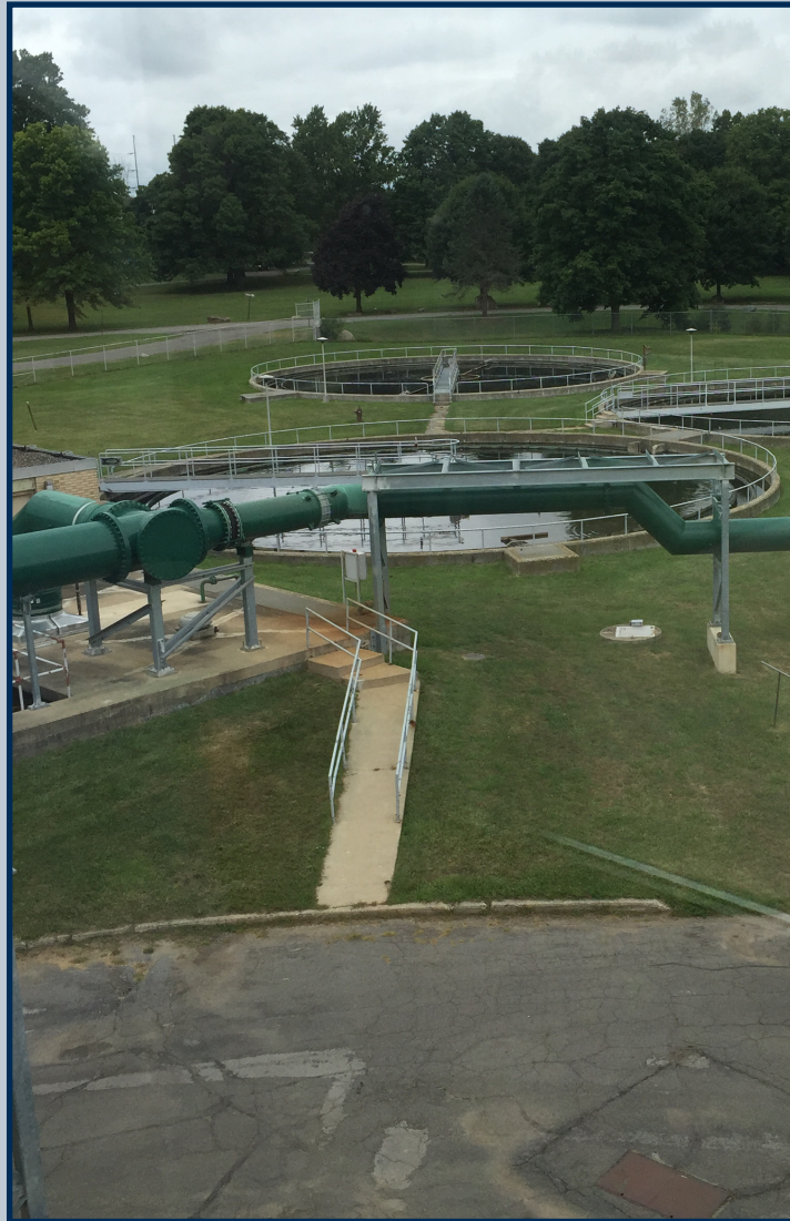
Settling tanks at the City's wastewater plant.
