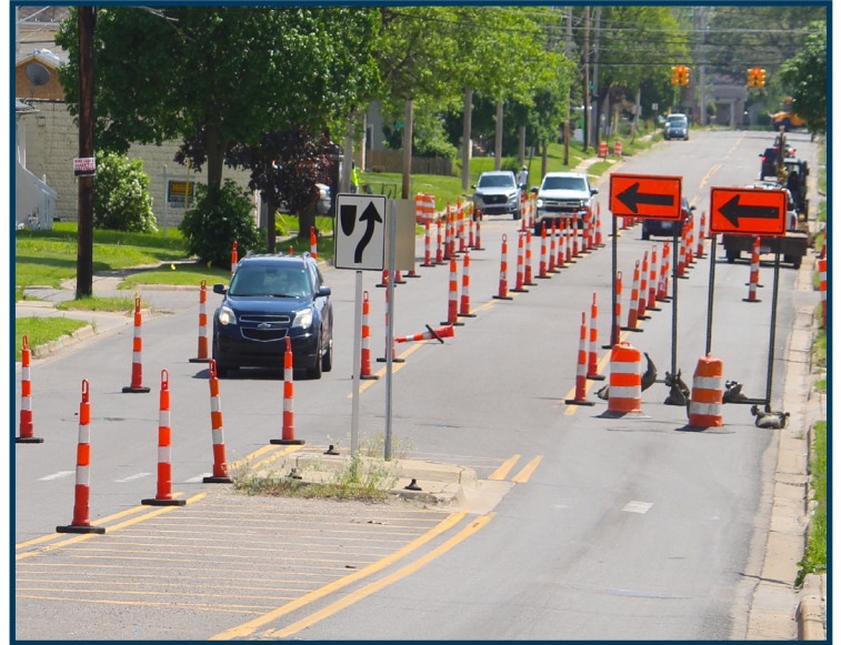
Lead service line replacements on S. MLK Drive in May 2024.
