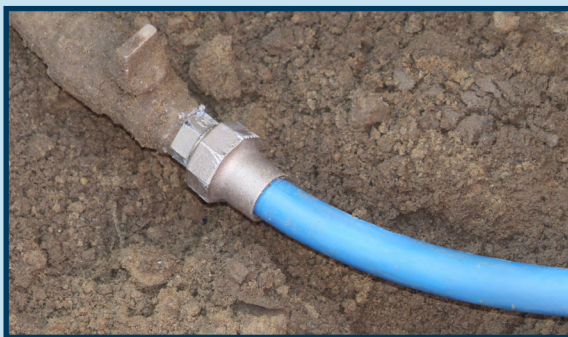
Lead service line replaced with new pipe.
