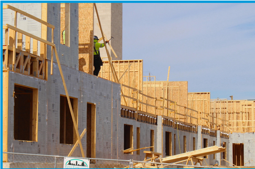
Construction underway at The Blackstone Apartments in Downtown Jackson.
