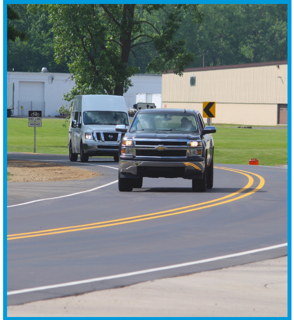
E. High Street reopens following resurfacing.
