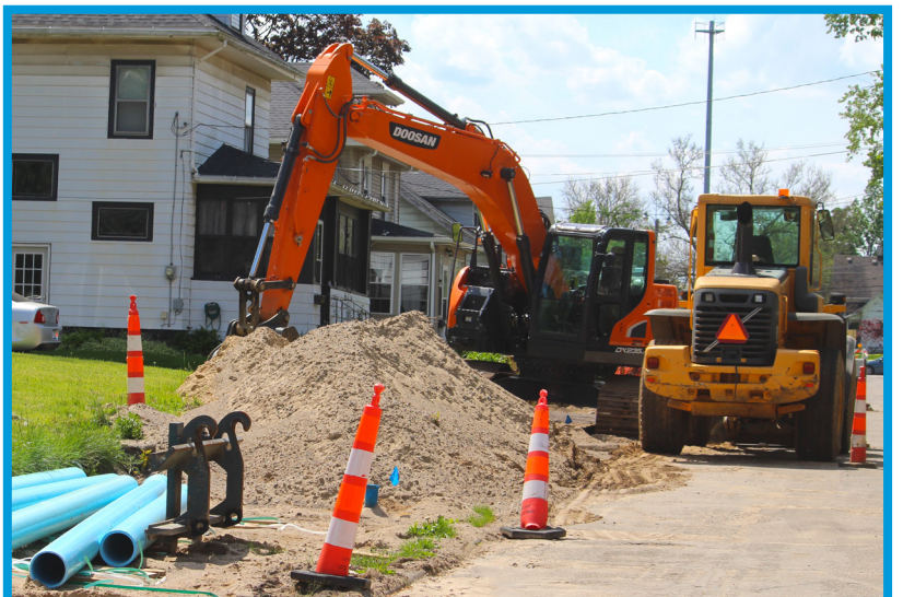
Water main replacement on Arnold Street.
