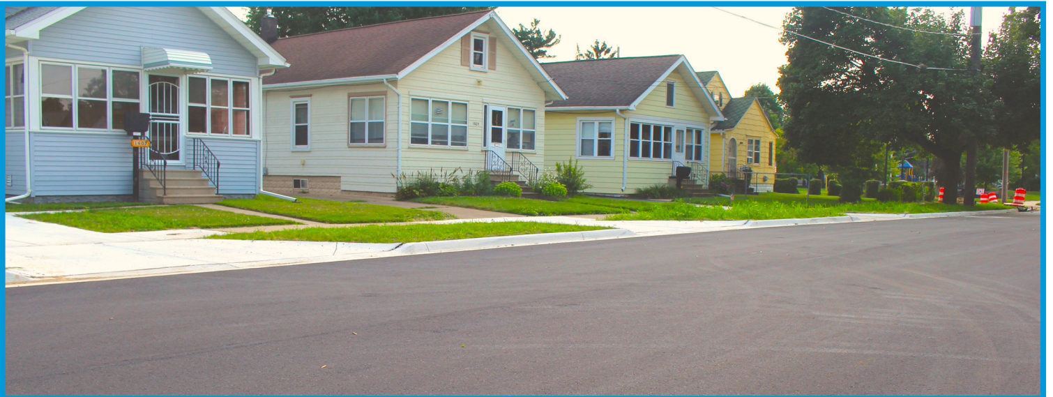
Reconstruction project complete on Blakely Avenue.
