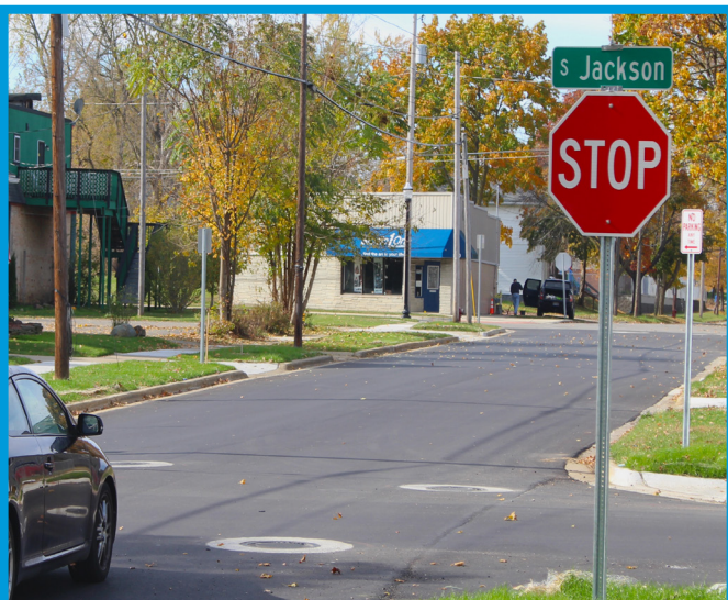
Construction project complete on W. Biddle Street.
