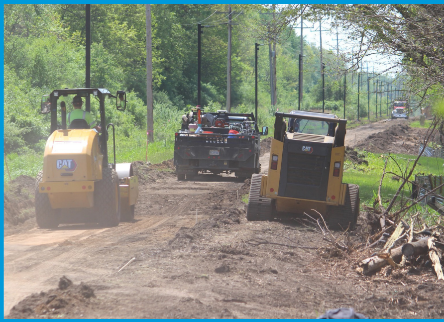
Construction underway on the MLK Equality Trail near S. West Avenue.
