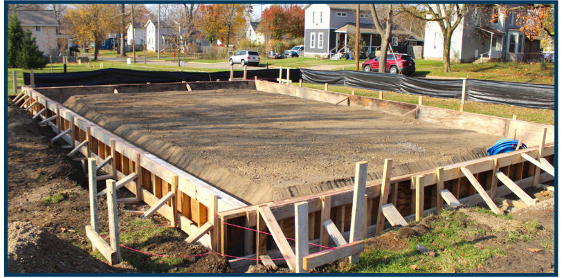
New house under construction on N. Perrine Street.
