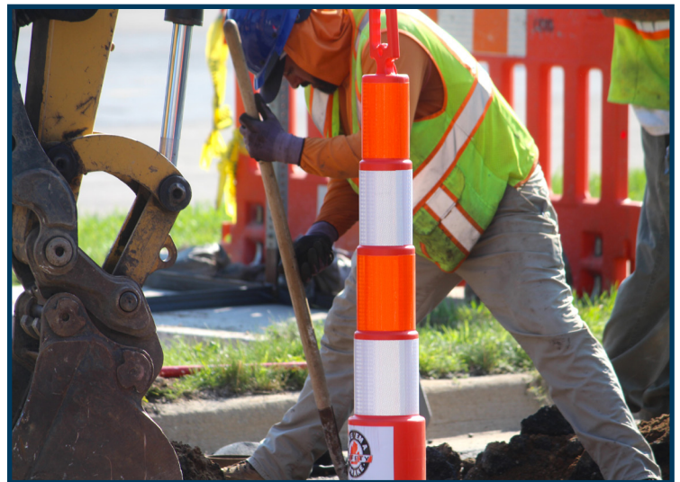
Construction worker repairs a Jackson street.
