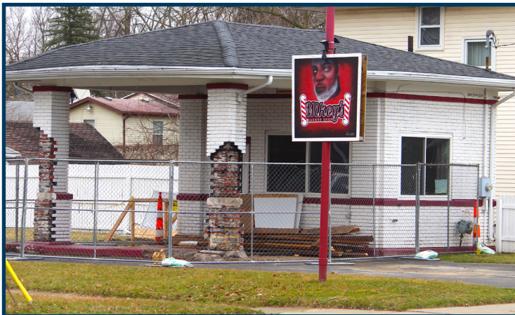
Renovation underway at Mikey's Barbershop on S. MLK Drive.
