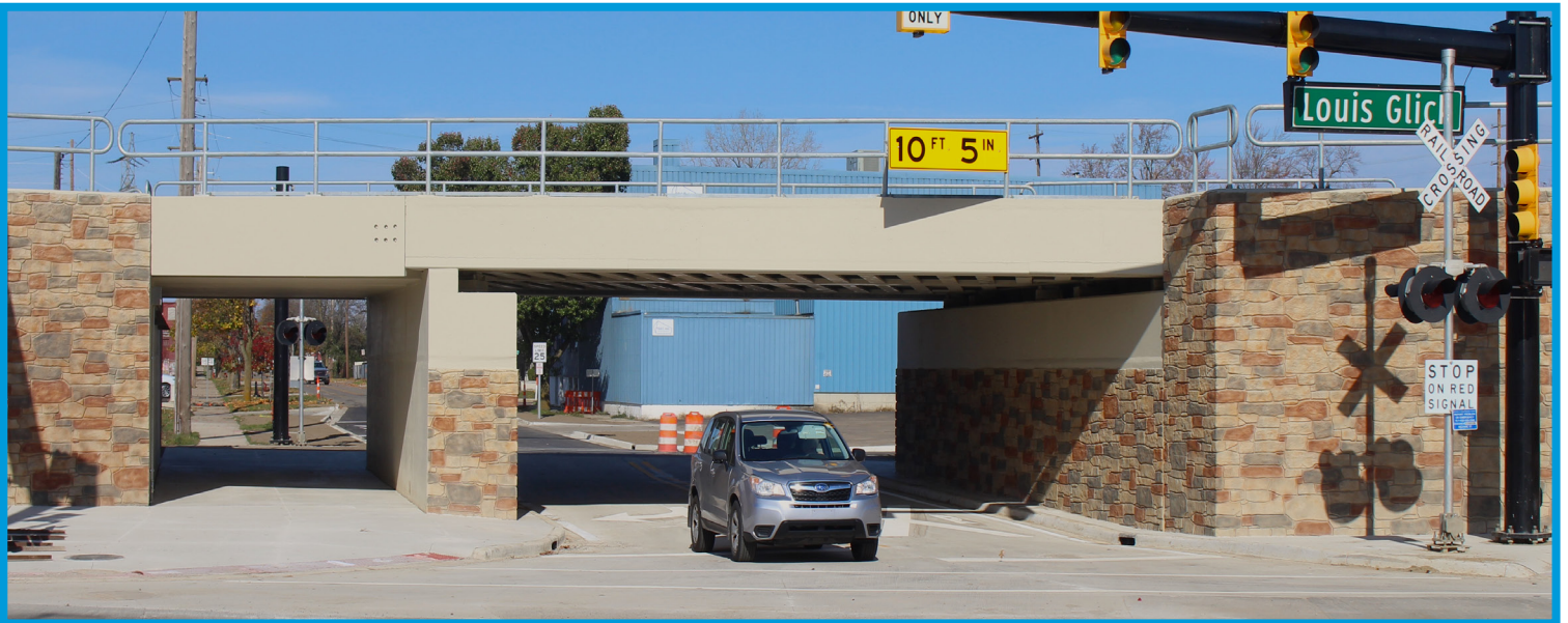
Railroad bridge replacements at N. Mechanic and N. Jackson streets were completed by MDOT in 2023.
