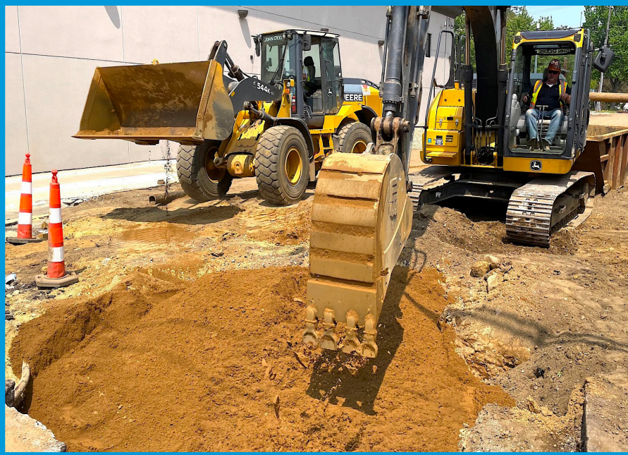
Construction underway on N. Perrine Street.
