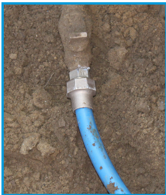
Updated water service line installed by DPW.
