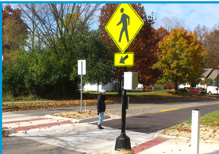
Trail crossings were made safer with new pedestrian signals.
