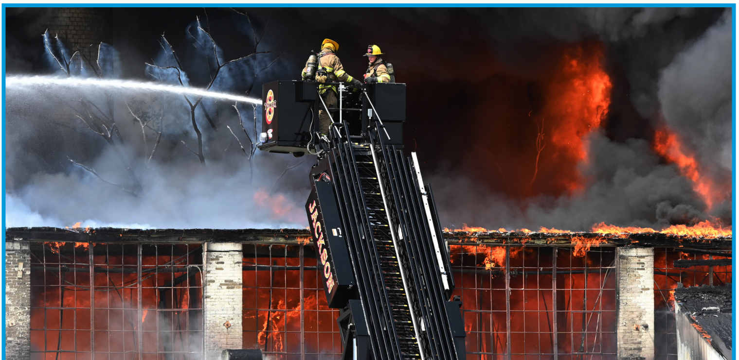
Jackson fire crews responded to a massive fire at a vacant industrial building on W. North Street in Aug.
