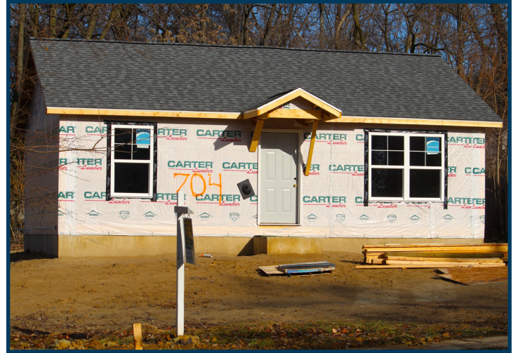
A new home under construction on W. Ganson Street.
