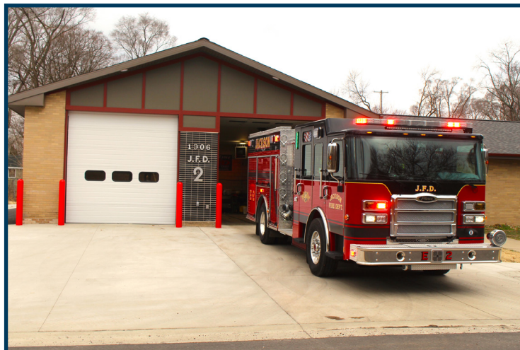
Fire Station No. 2 on S. Milwaukee Avenue.
