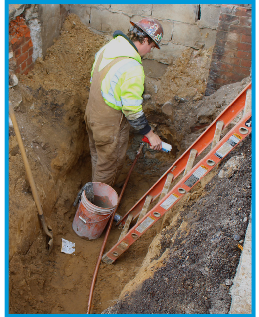
Lead line replacement on E. Michigan Ave.
