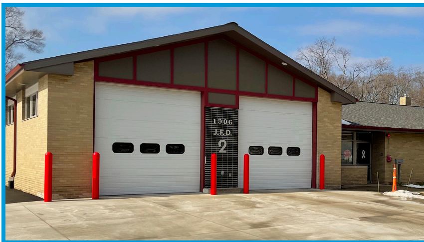
Fire Station No. 2 reopened in 2022 and received a substantial renovation.
