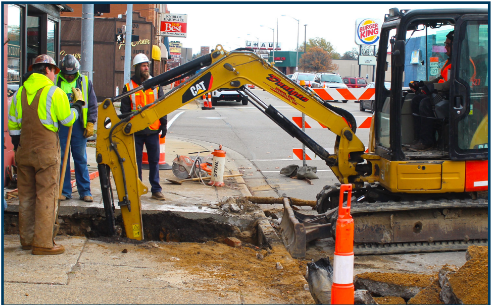
Lead service line replacements on E. Michigan Avenue in Nov.
