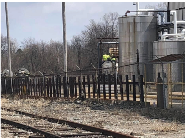
Carbon Dioxide leak in Leoni Township
