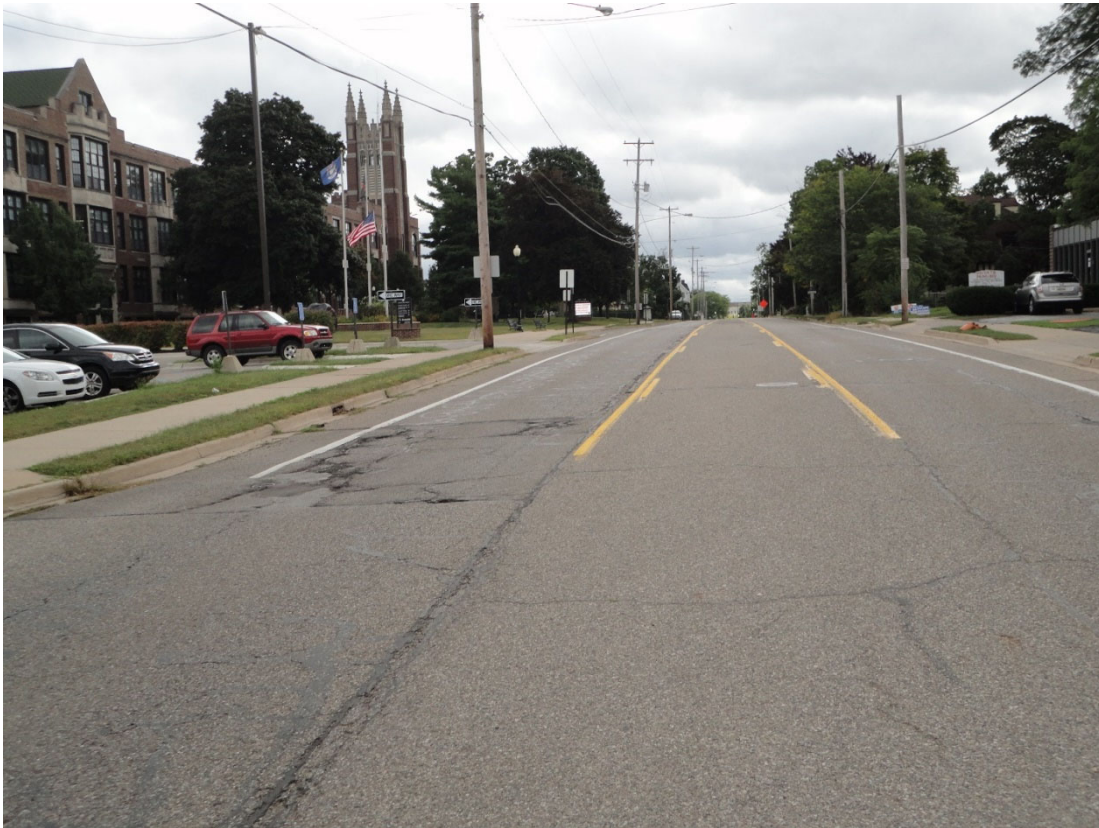
Photo 3: Wildwood looking east from Edward Street
