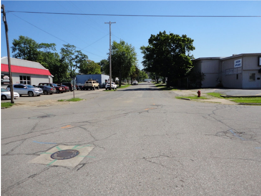
Photo 3: Pearl Street at Park Avenue looking east
