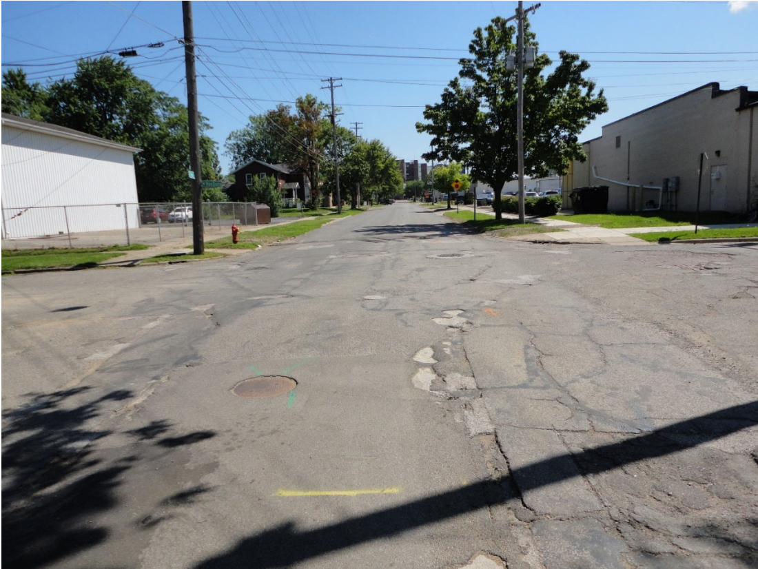
Photo 5: Pearl Street at Van Dorn looking east
