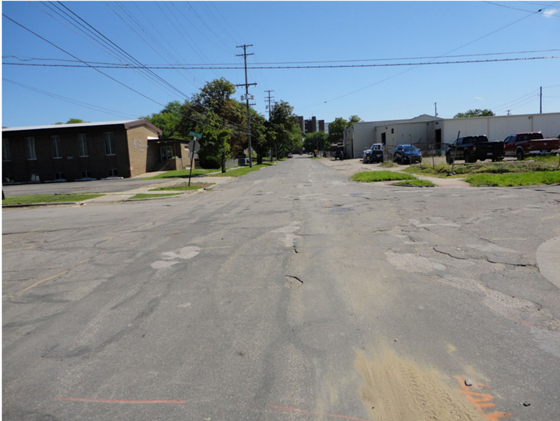
Photo 7: Pearl Street at Perrine looking east
