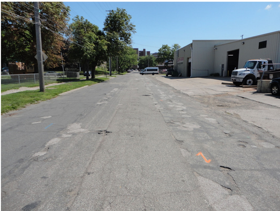
Photo 8: Pearl Street between Perrine and State looking east
