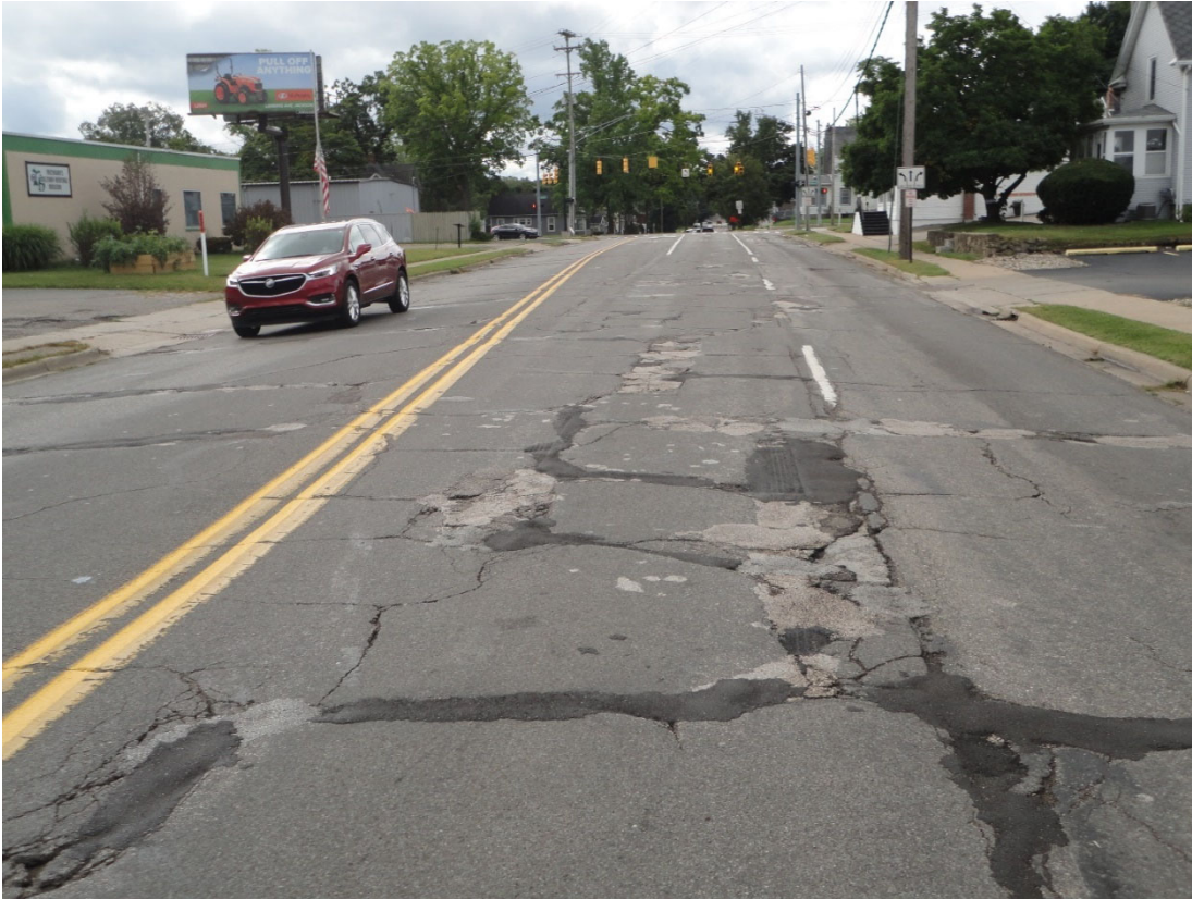
Photo 1: Wisner Street looking south from in front of 315 N. Wisner Street
