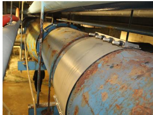
Figure 4-4 - Repair clamp on 24-inch filter backwash supply.
