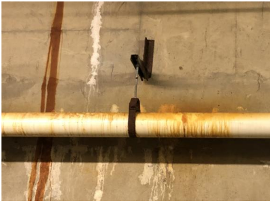
Figure 6-2 - Typical surface wash pipe support.
