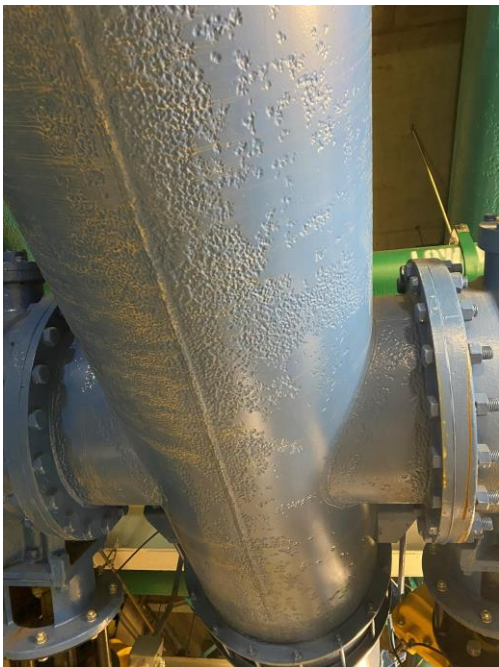
Figure 4-8 - Fifty-year-old steel piping was restored at the Muskegon WFP in 2004.
