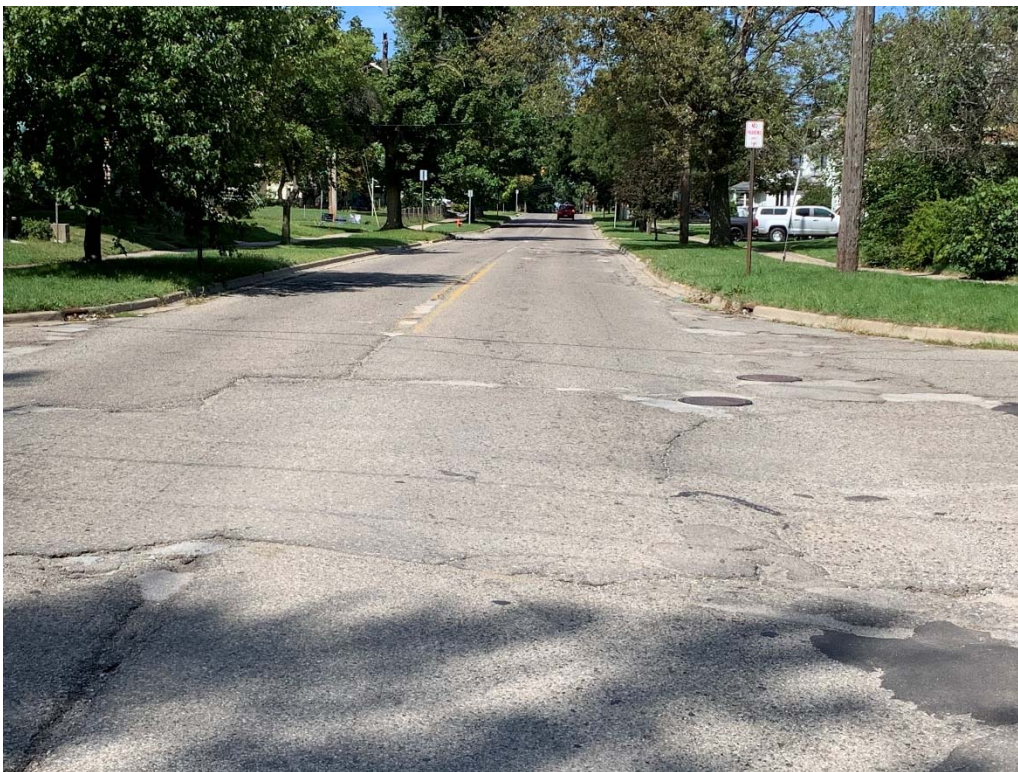
Photo 2: Steward Avenue, at Trail Street facing north
