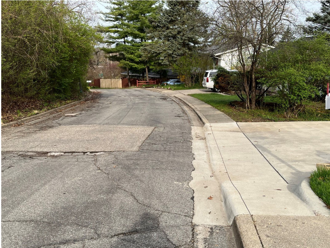
Photo 1: Oakridge Drive from west of Grovedale facing west
