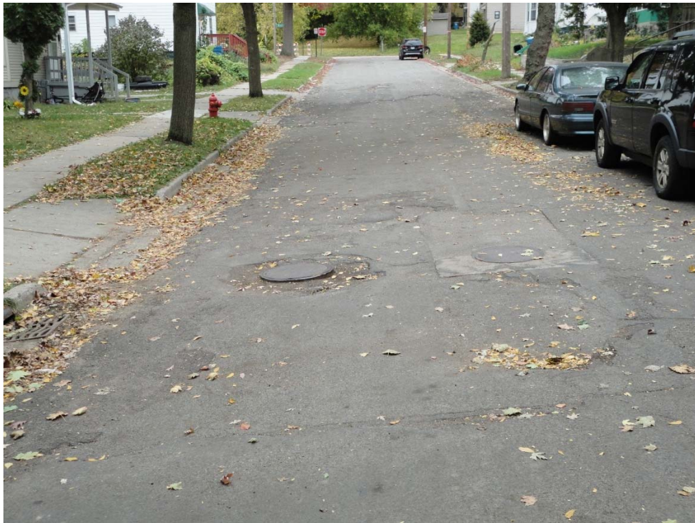
Photo 2: Cooley Place at 807 Cooley, looking south.
