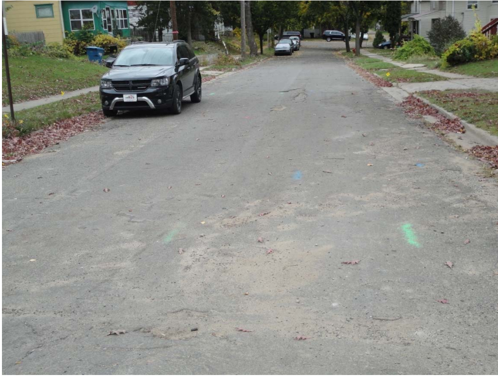
Photo 3: Cooley Place at Morrell Street, looking north.
