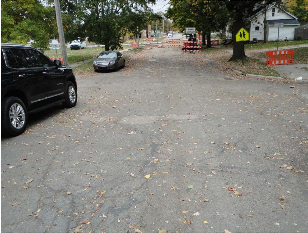
Photo 3: Biddle Street at Cooley Place, looking east.
