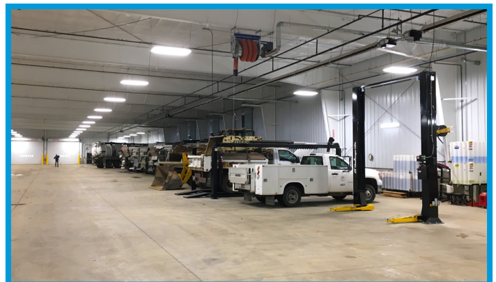
The new DPW Operations Center was completed in fall 2020.
