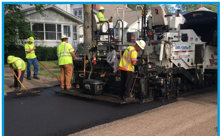
Resurfacing on N. Higby Street.
