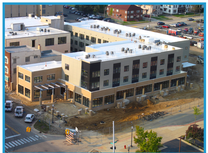
The Albert Kahn Apartments under construction on S. Jackson Street.
