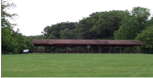
The Picnic Shelter holds about 100 people and is approximately 28 x 50.
